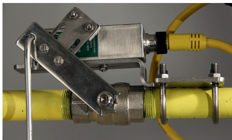
Figure 3: Safety Shower Valve in Activated Position
